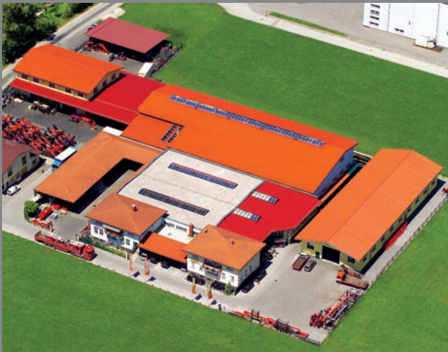
In the workshop in Elsbethen near Salzburg EPSILON ON Road, OFF Road and Recycling cranes as well as STEPA farm, mobile and Tractor cranes are produced.
