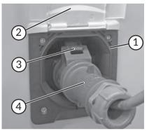
Connected 230 V feeder plug Supply via mains connection
